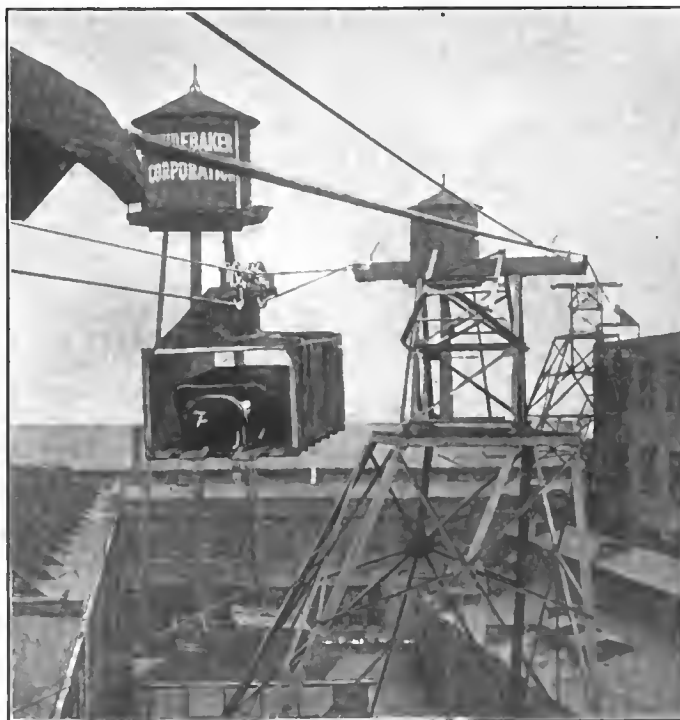
New aerial conveyor system installed by the Studebaker Corp., Detroit, for the transfer of bodies and wheels from the finishing department to the assembly floor, a distance of 780 feet. Steel cables carry the load, and they are supported by trestles, with the longest span 178 feet
